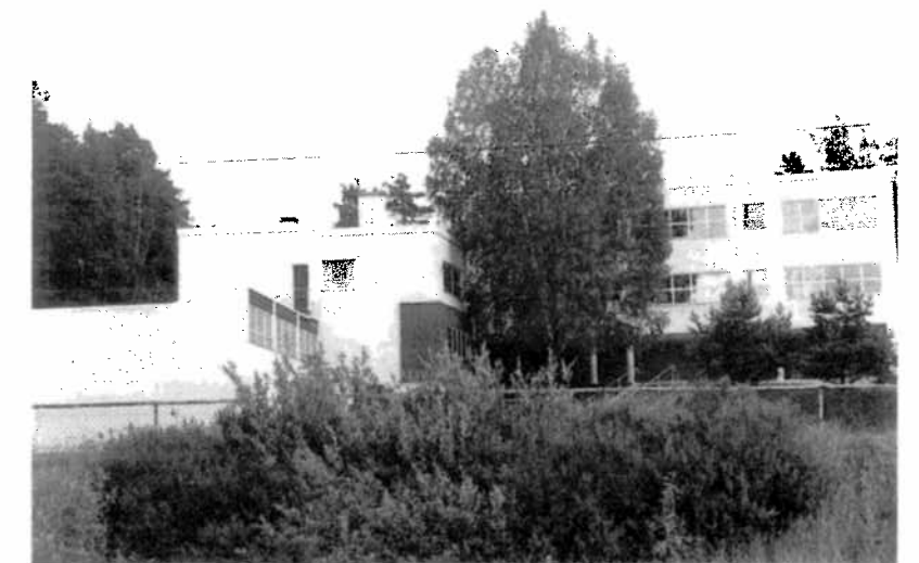
Figure 1.1c View towards double height entrance hall with the main classroom block on the right.
