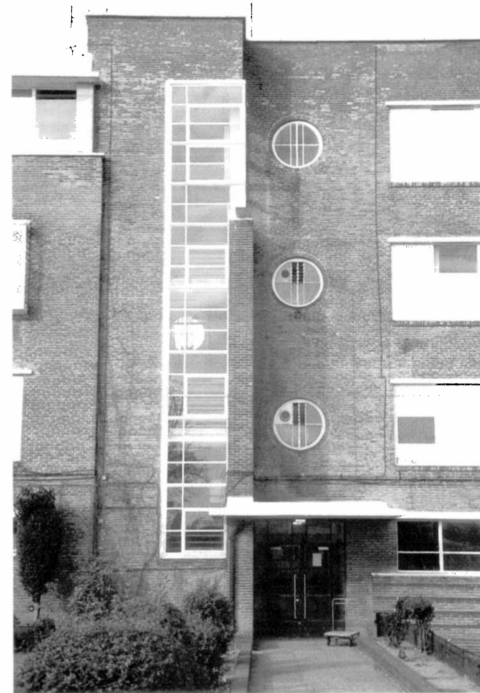
Figure 1.18 Burlington Secondary School (1935), London, by Burnet Tait and Lorne. (Photo: © Mark Dudek.)
