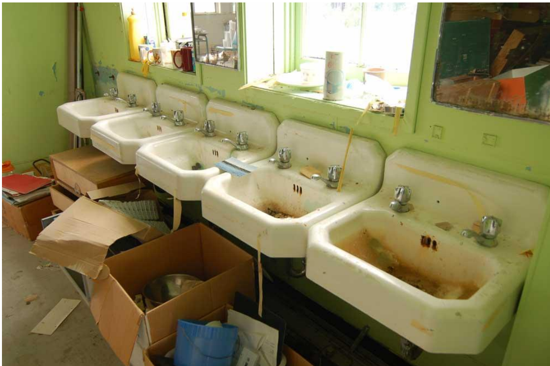
Figure 4. 18 - St Michael's Indian Residential School, Alert Bay, BC. Sinks in Boys Dormitory. Photo: Geoffrey Carr (2009).
