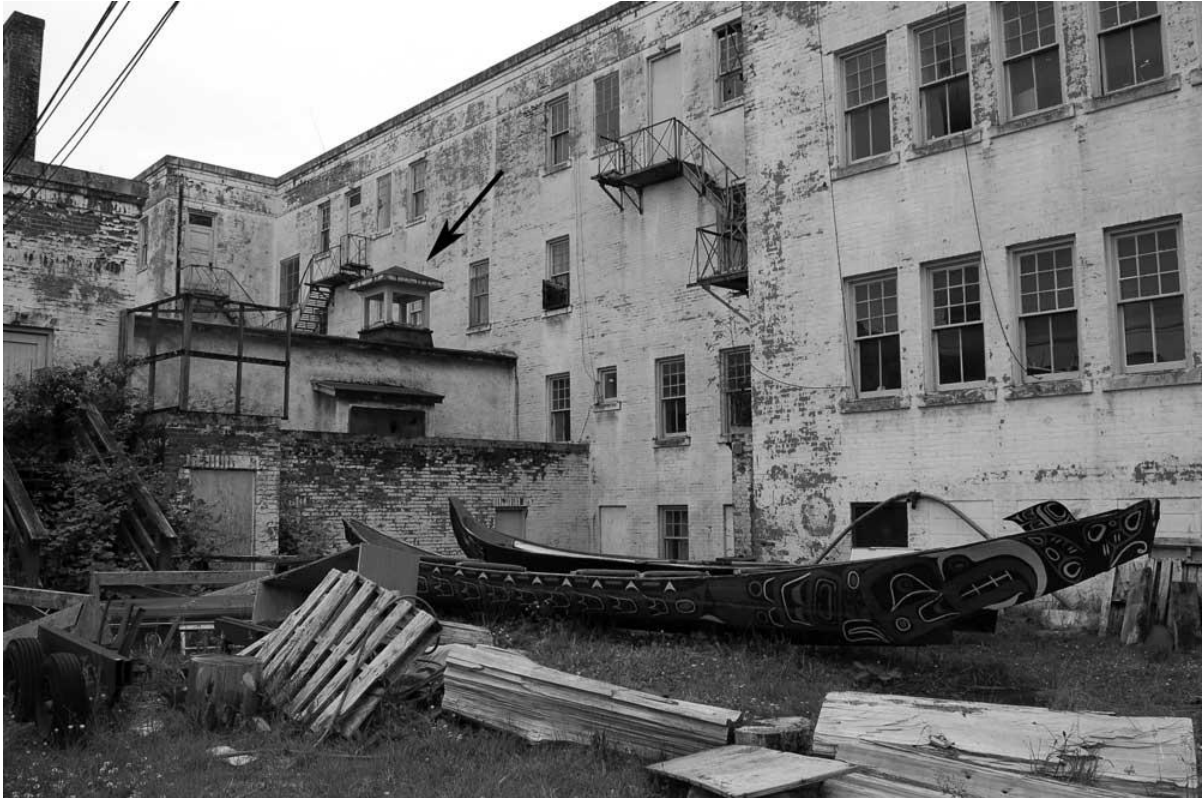
Figure 3. 2 - St. Michael's Indian Residential School, Alert Bay, BC. Small bell tower atop corridor between main building and chapel (assembly hall). Photo: Geoffrey Carr (2009). Arrow indicates tower.
