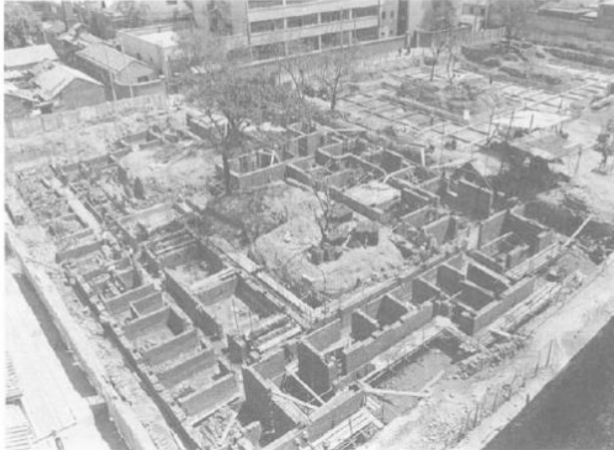
Figure 6. Foundation work, showing the efforts to preserve existing trees, to which original residents have emotional ties. (From Wu, Liangyong. 1999. Rehabilitating the Old City of Beijing )
