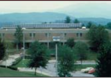
This roof-mounted solar system was installed by vocational education students at McDowell High School.
