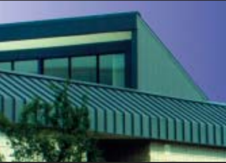
Clear double glazing has to be used to optimize solar access. Overhangs block excessive radiation in the warmer months.
