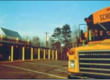
Photovoltaic systems in schools provide substantial energy savings and are educational tools for sustainability.
