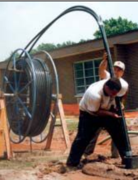
Photo: Advanced Energy
