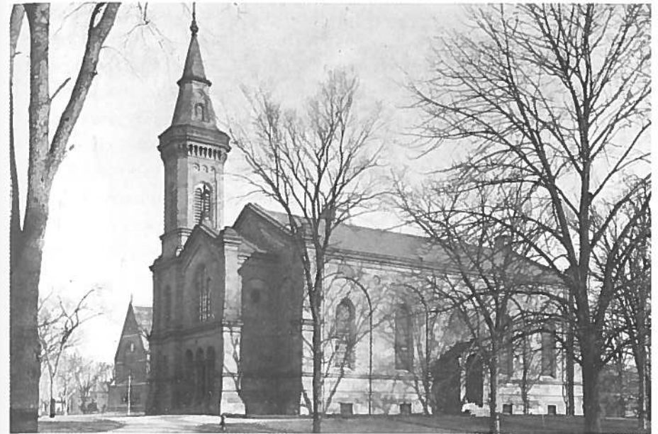
Figure 3.4. View of the southern elevation of Appleton Chapel (1853) facing Widener Library. Courtesy of Harvard University Archives, HUV 53 (1–1a).
