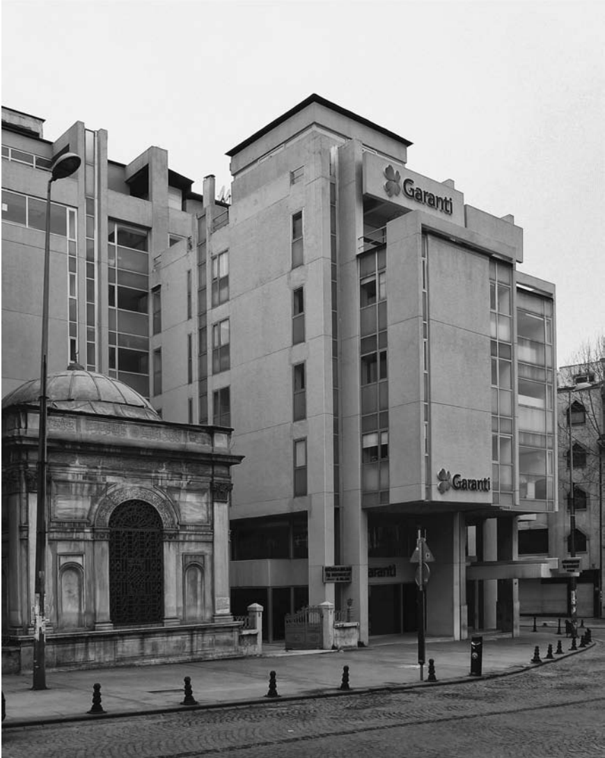
Figure 8.5 Contemporary photograph of the Istanbul Reklam Building, 2014. Aykut Köksal's photograph
